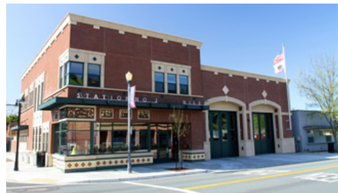
LEED™ Silver-certified Fire Station #2—Niles Boulevard
